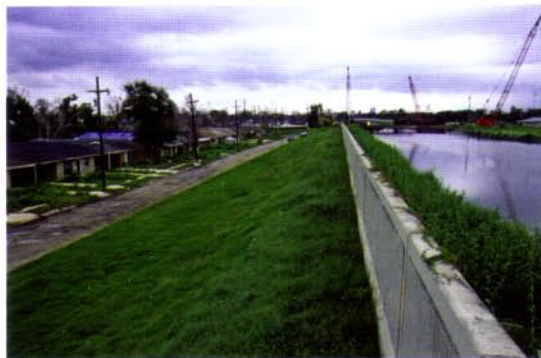
Fig. 8. An intact section of levee along the London Avenue Canal holding back water that stands well above the houses—which were flooded when water swirled round from a levee break below the distant crane on the left.
