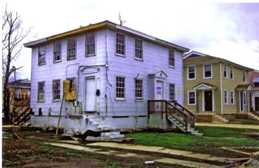
Fig. 13. A Gentilly house built on a piled box that now stands about 150 mm clear of the ground that has subsided, with a very visible gap through the broken steps.
