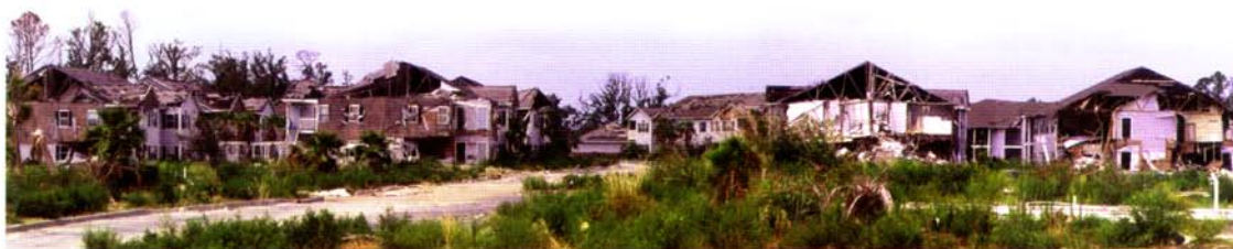
Fig. 15. The storm surge through the ground floors and wind damage to the upper floors, wrecked an estate of new houses in from the shore near Gulfport.
