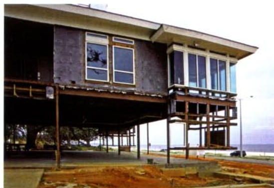
Fig. 13. A Gentilly house built on a piled box that now stands about 150 mm clear of the ground that has subsided, with a very visible gap through the broken steps.
