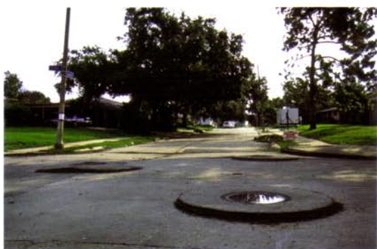
Fig. 12. In a Gentilly road near the London Avenue Canal, drain rings stand 50 mm above the subsided tarmac around them.
