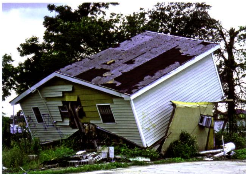
Fig. 11. A two-storey Lakeview house that lost most of its ground floor to the flood surge.
