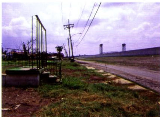
Fig. 10. The newly rebuilt levee along the Industrial Canal rises above a part of the Ninth Ward that was stripped of its houses by the inrush of water, except for the concrete steps that once led to a front veranda.
