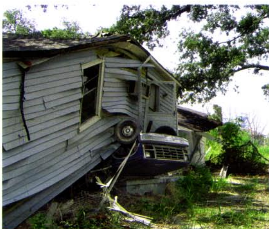
Fig. 9. Close to the levee break in the Ninth Ward, a timber house floated off its footings, to land on an upturned car that was already on the foundation slab of another house.
